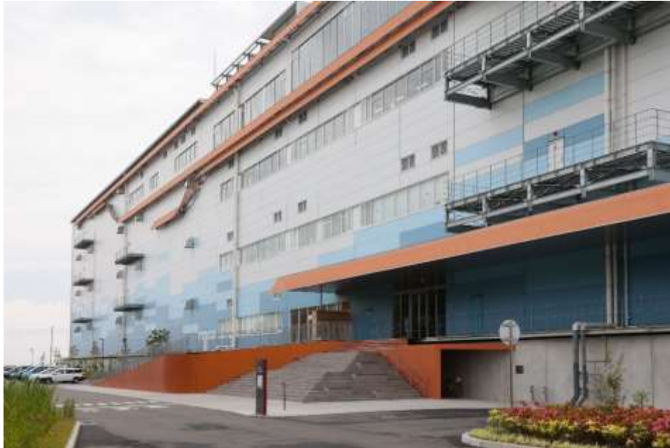
The new Sachiura Parts Center located in Sachiura, Yokohama
