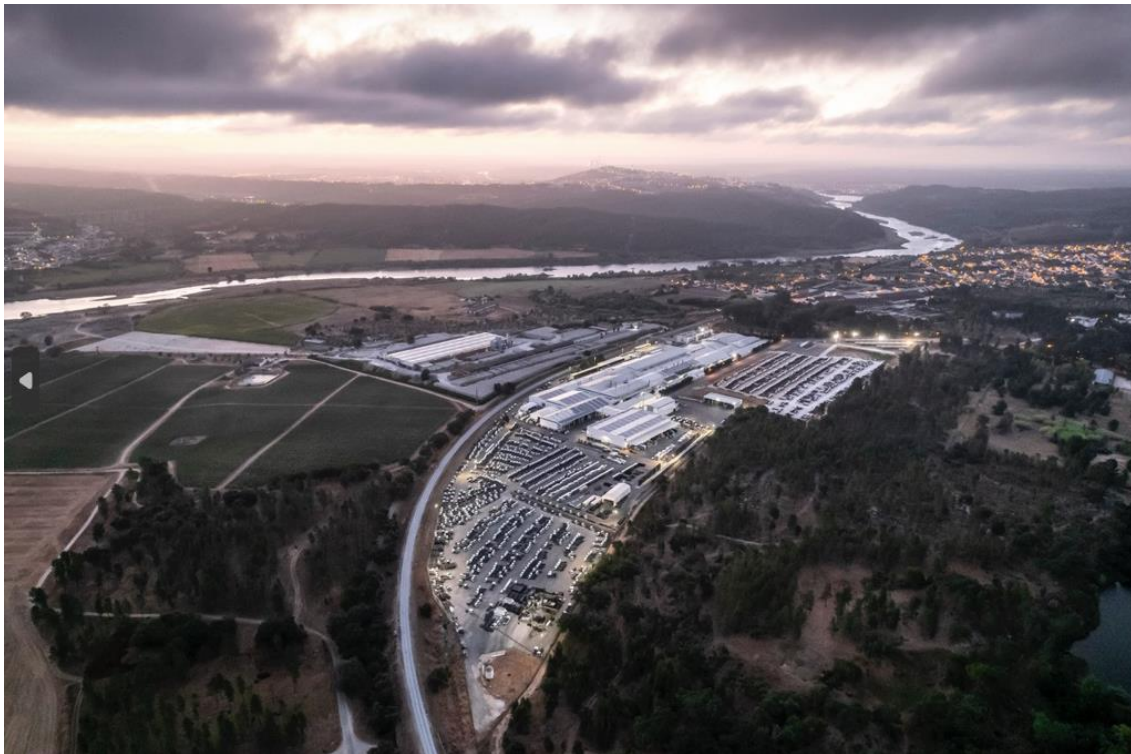
A bird's-eye view of the Tramagal Plant
