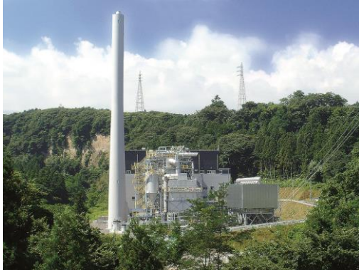
ORIX's Agatsuma Biomass Power Plant
